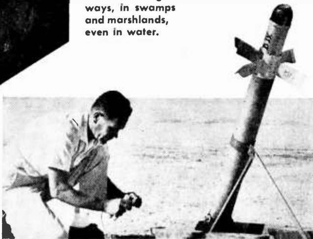
Ping Pong , a photo-reconnaissance missile developed by Lockheed, returns to launch area after flight that includes mid-air stop and "bounce-back."
